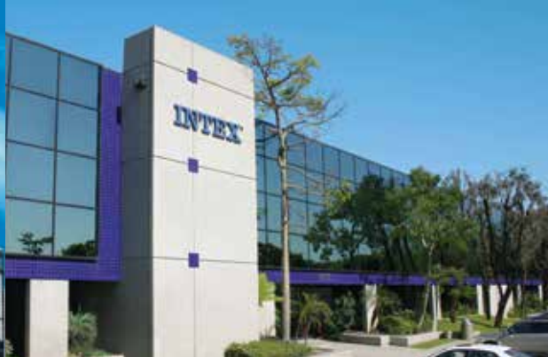
Intex Recreation Corp, Long Beach, CA, USA
